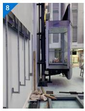
The lift car was then assembled and installed, including bespoke lights, gold canopy and glass walls
