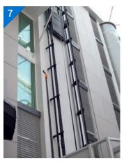
The lift guides are then installed on which the bridal lift will travel between the ground and first floors
