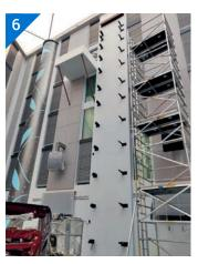
Scaffolding is erected to allow the guide fixing brackets to be fitted up the full travel height of the lift
