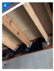
On-site building work exposed the lower level ceiling so a hole could be cut out to allow construction of the platform lift shaft
