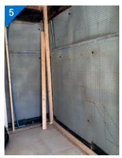
The staircase was removed and the lift shaft was built to overcome the issue of insufficient head room for the chosen model
