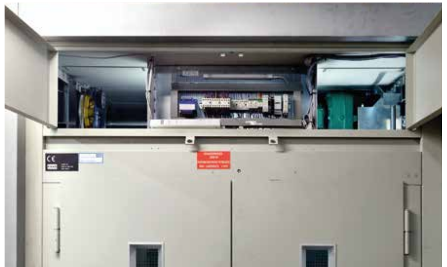
Access to controller above top landing doors. Installation comes complete with aluminium access ladder
