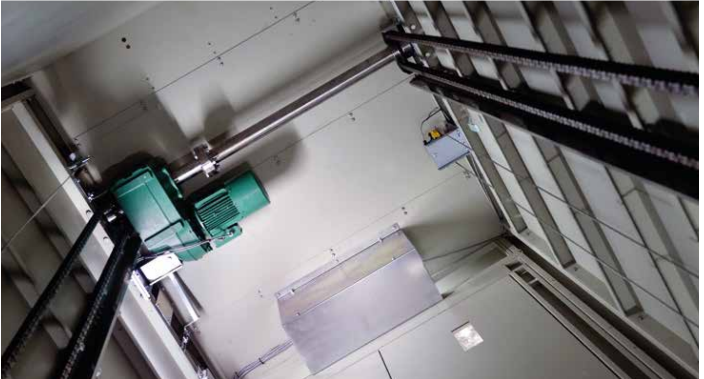
Motor and twin heavy duty chain drive system
