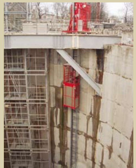
This Stros BV 400 hoist has 400 kg of lift capacity.
