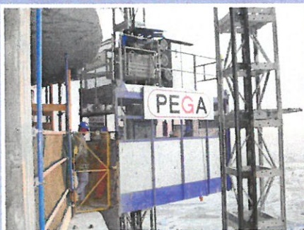
One of the main Pega hoists on the tower, showing the landing arrangement and the strengthened tower sections.
