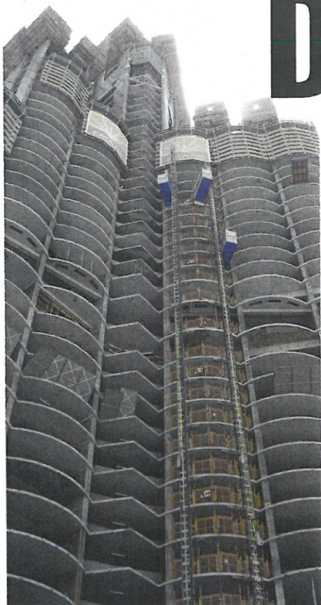
One of the main Pega hoists on the tower, showing the landing arrangement and the strengthened tower sections.
